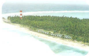
100 KWp SPV power plant at Kiltan Island, Lakshadweep
